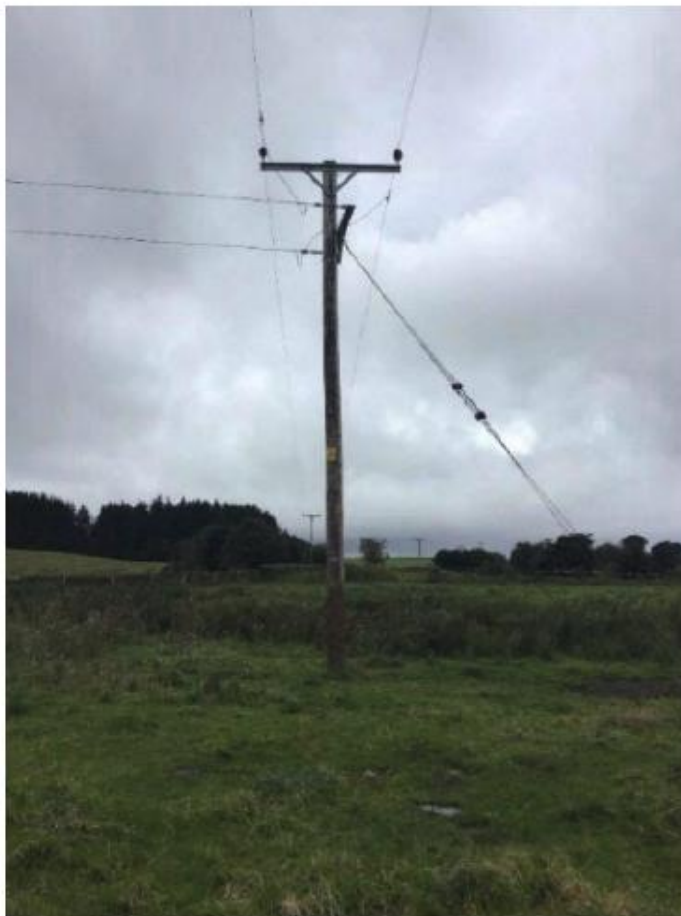
Figure 8: (Left) A 33 kV two-phase overhead line (Right) A 20 kV three-phase overhead line
