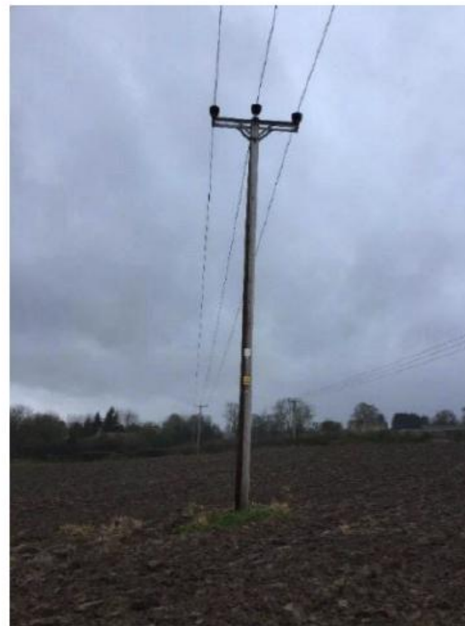
Figure 8: (Left) A 33 kV two-phase overhead line (Right) A 20 kV three-phase overhead line
